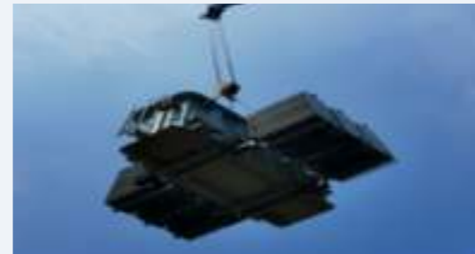
Replacement of Energy-Saving Transformers
